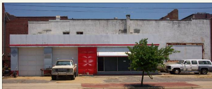
Historic Station Today
