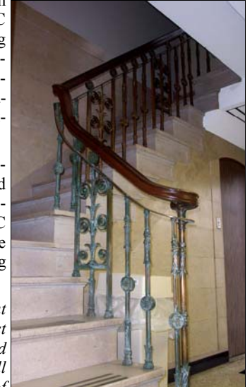
Original Staircase from First Floor to Second.
