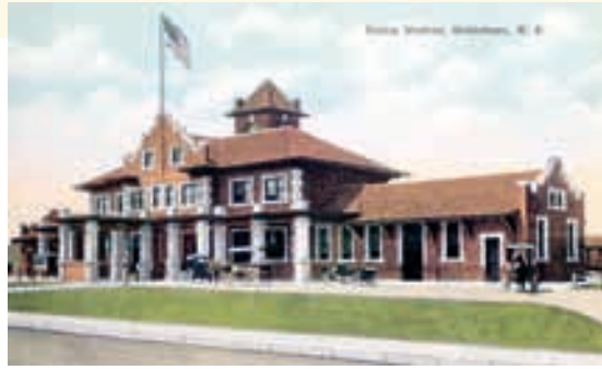
The historic Union Depot in Goldsboro has been purchased for restoration as a multi-modal transportation facility.
