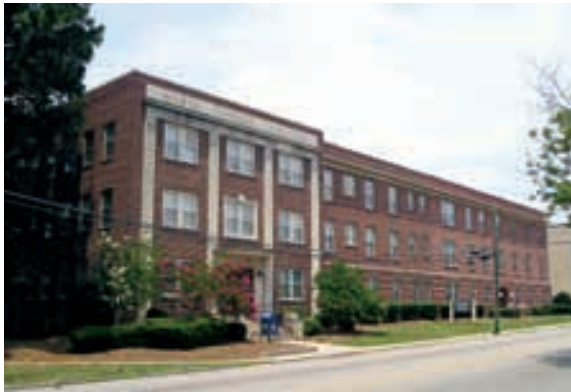
Maria Parham Apartments (formerly Maria Parham Hospital), Henderson, Vance Co.
